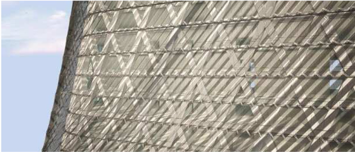
Architecture dominates the Design and Computation gallery at SIGGRAPH 2008. The Phare Tower, La Défense by Marte Doscher and Satoru Sugihara uses computational design for the "diagrid" of the structure. All images ACM SIGGRAPH 2008.
